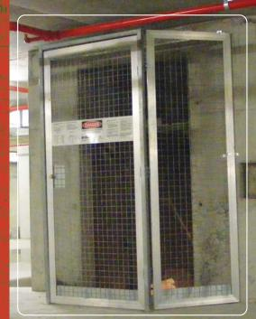
Aztex Liftwell Screens give you peace-of-mind on site. They weigh only 40 kg—over 40% lighter than conventional steel screens, while being structurally strong and robust.
